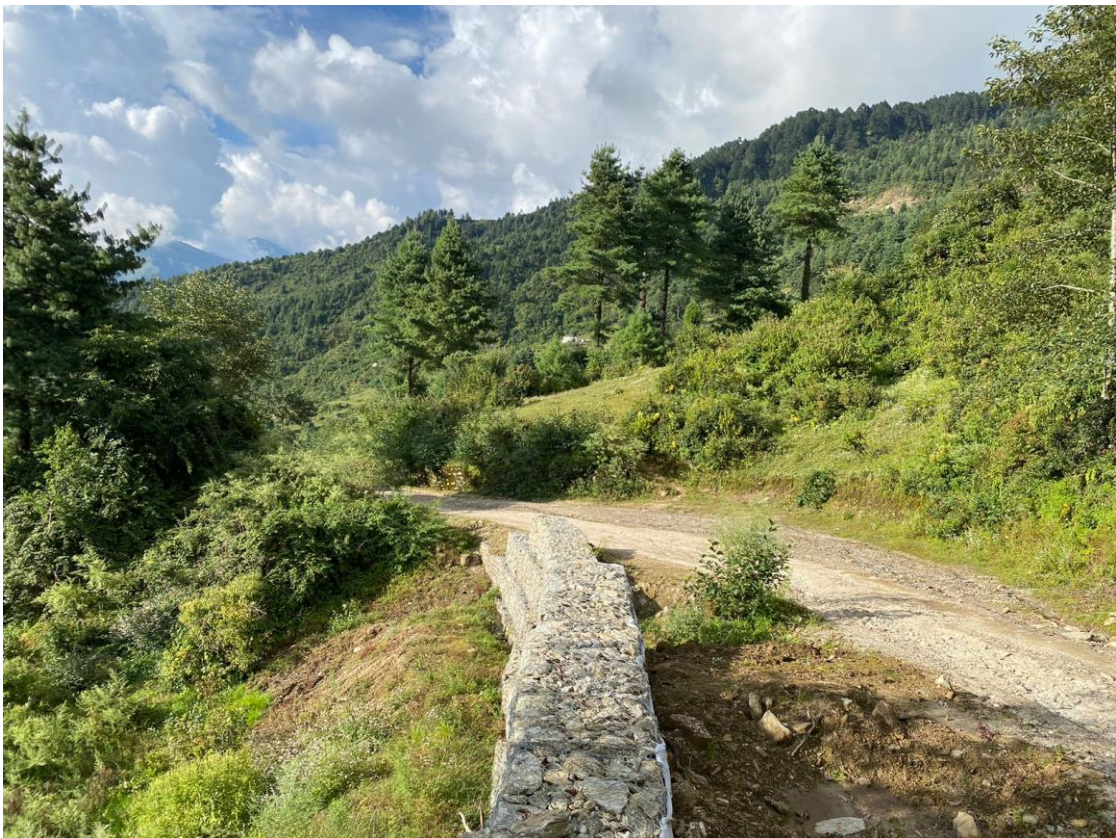
Figure 13 The Photo of the Site during the survey
